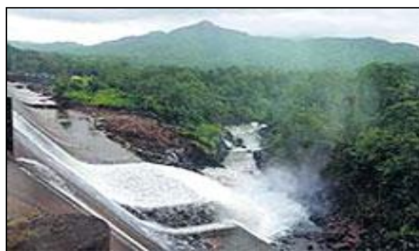
Picture No. 2-1: Vaitarna Dam
