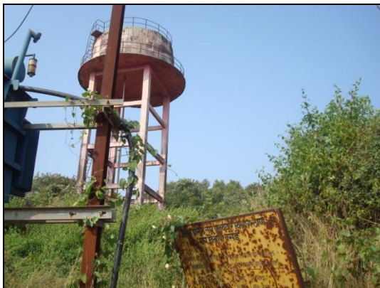
Picture No. 2-21: Overhead water tank near Netaji Lake
