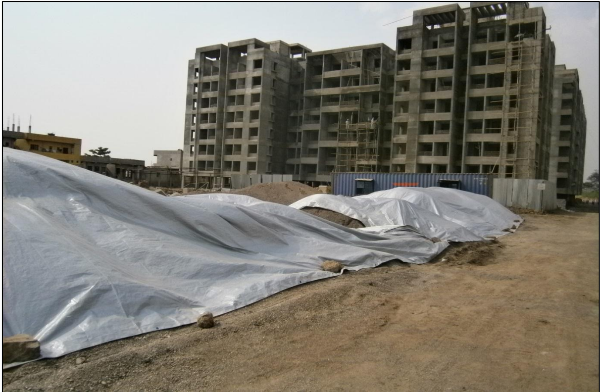
Picture No. 3-1: Covering of sand at a construction site
