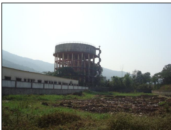
Picture No. 2-23: Overhead water filtration tank
