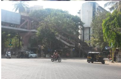
Existing Stairs to FOB
