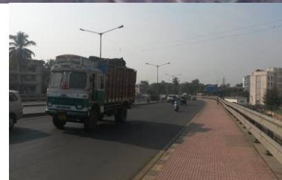
Flyover next to Station Building
