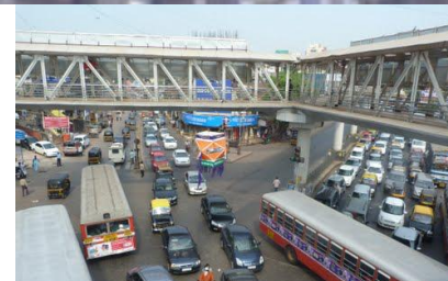
FOB at junction near station end
