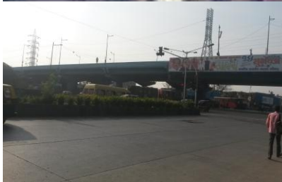
EEH with Empty lot in the foreground
