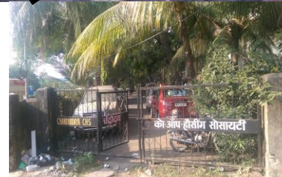
Location for Entry Structure
