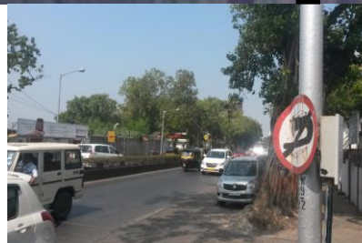
Juhu Airport Boundary Wall
