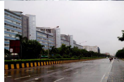
Existing 14.0m carriageway
