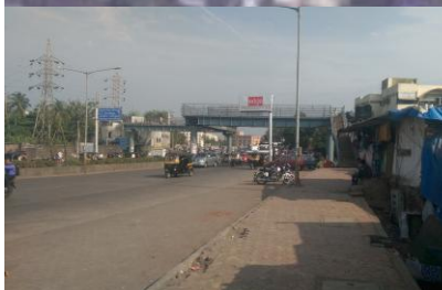
Existing FOB at Station Location
