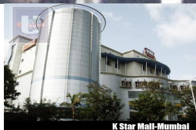
Mall near Station Entry
