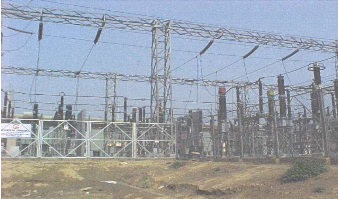
Typical High Voltage Receiving Sub-station
