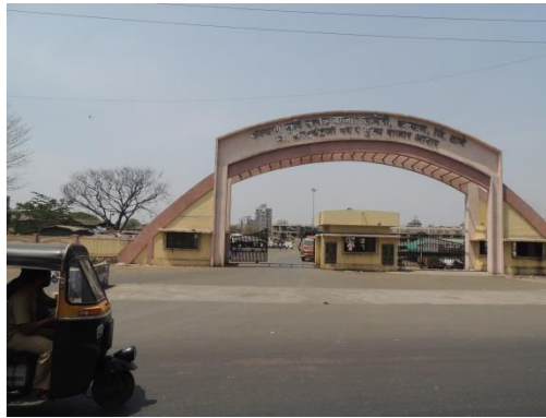
Figure 7.4: Kalyan APMC Metro Station
