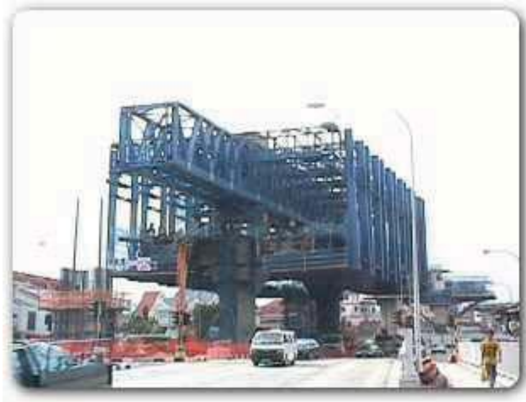
Figure 6.9: Pre-cast segmental box girder
